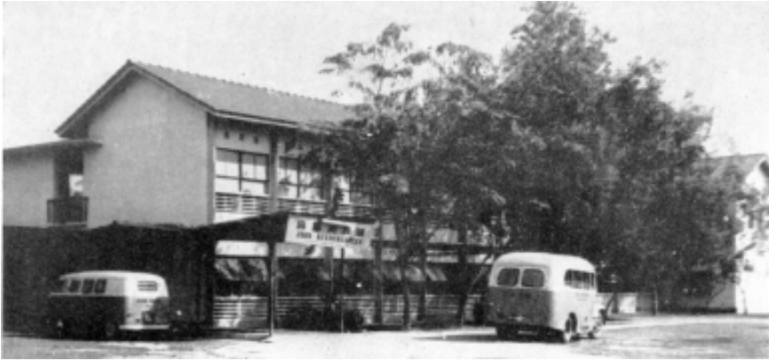
Zion Kindergarten's Original Building
